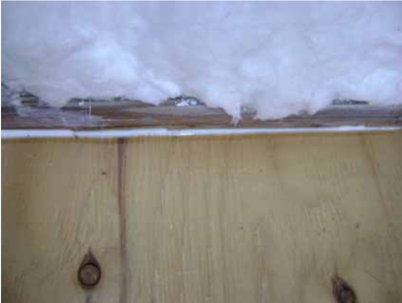
Caulking The Bottom Plate
